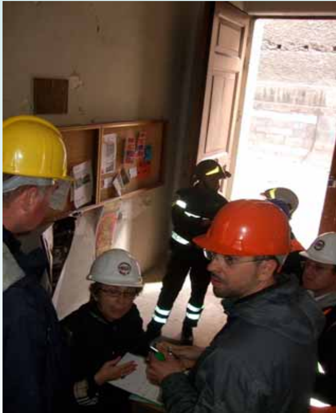
a joint team assessing the state of damage of an historical building in l'Aquila
